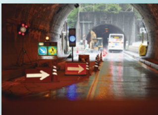
Service and utility tunnels, construction sites
